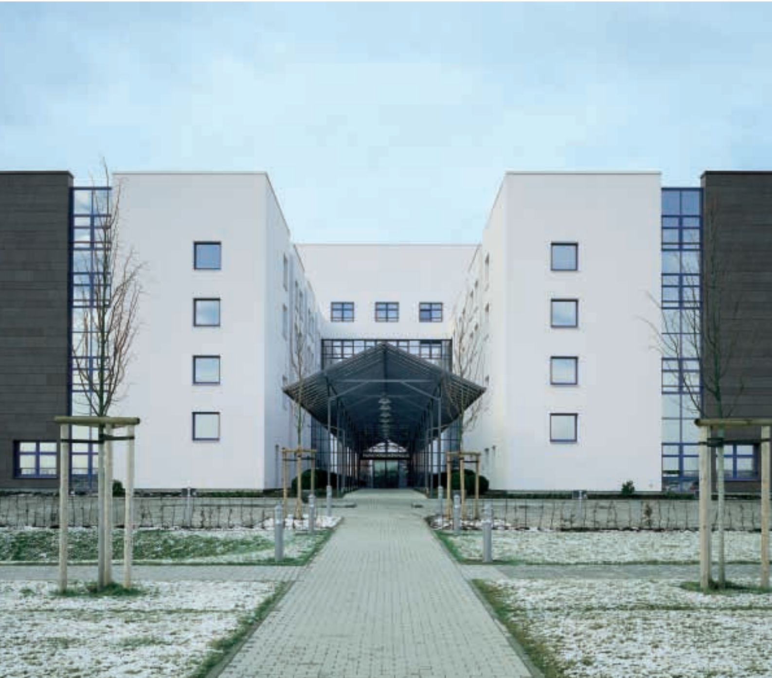
Park-Krankenhaus, Somatic Clinic, new building.
